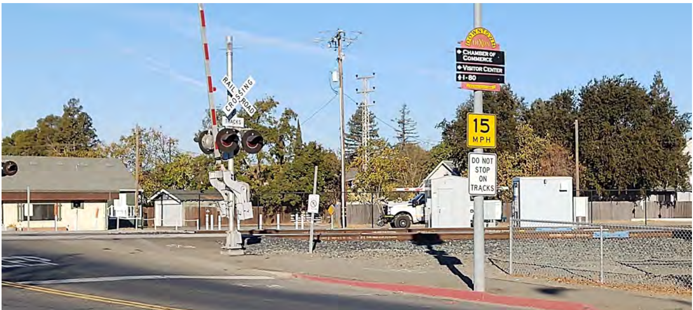
FIGURE 5: STEEP APPROACH AT EAST A STREET CROSSING
