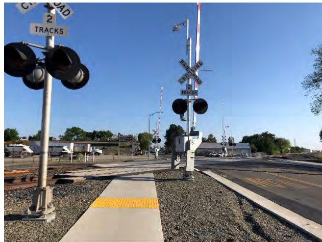
Figure 4 – 1 st Street Existing Conditions (April 2021)
