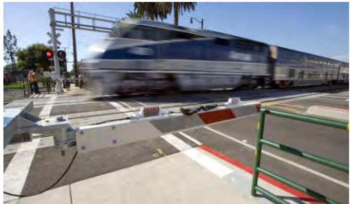
FIGURE 6. EXAMPLE OF A PEDESTRIAN GATE ARM APPLICATION (PALM AVE CROSSING, ORANGE CA)
