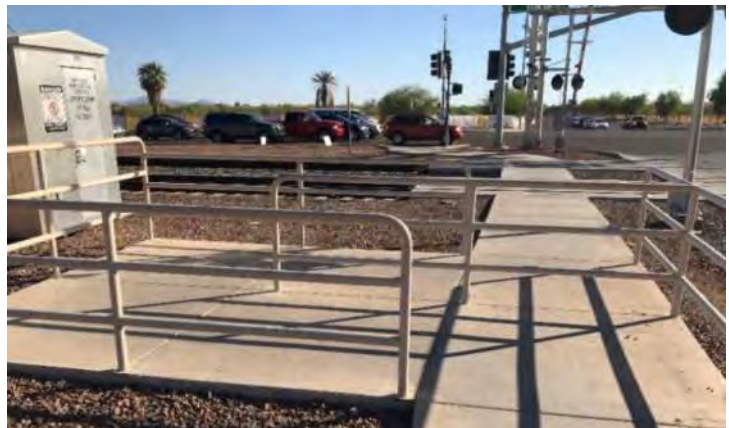
FIGURE 5. EXAMPLE OF A PEDESTRIAN BARRIER APPLICATION (BNSF COTTON CROSSING, PEORIA AZ)
