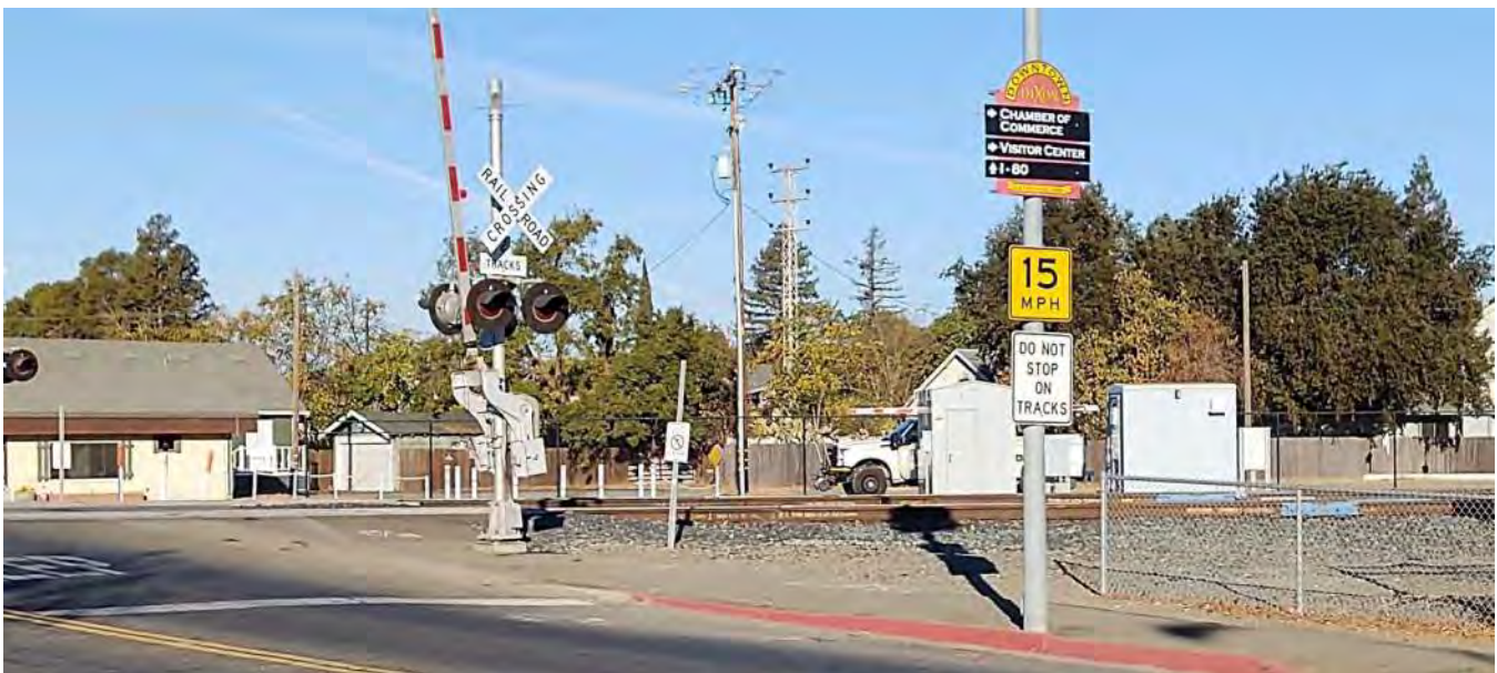
FIGURE 7. STEEP APPROACH AT A STREET RAILROAD CROSSING (LOOKING WEST)
